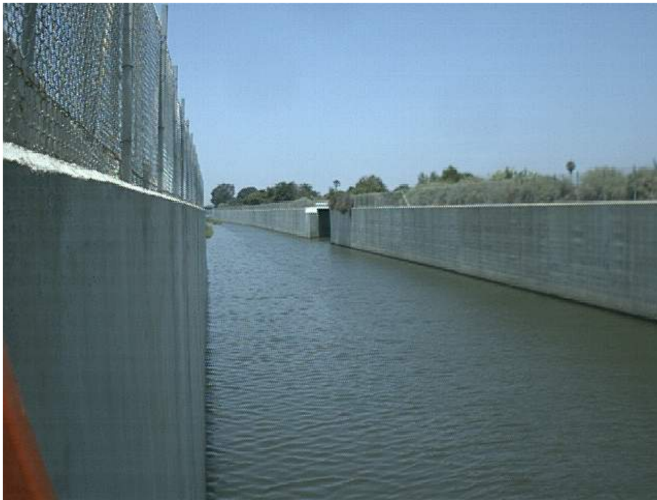
Figure 2 Upstream view of Greenville Banning Channel at Confluence with Fairview Channel
