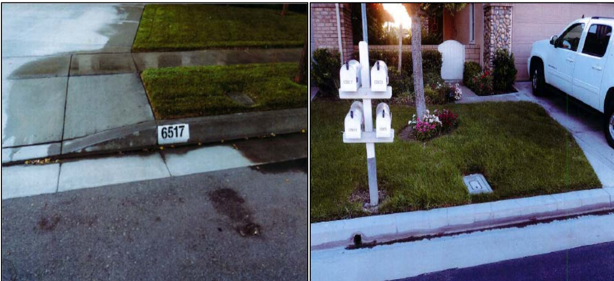
Figure 1 Typical irrigation excess runoff from front yards (a) and back yards via an underdrain (b) Photo credit: Ruben Valdez
