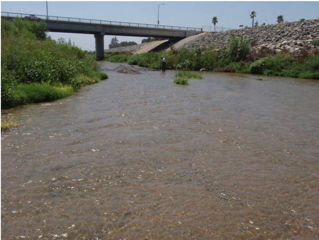
Figure 2. Site 1, Mission Blvd., the broader of the two channels at site.
