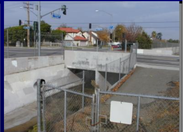
Cypress Channel @ Shaffer Ave (S6)
