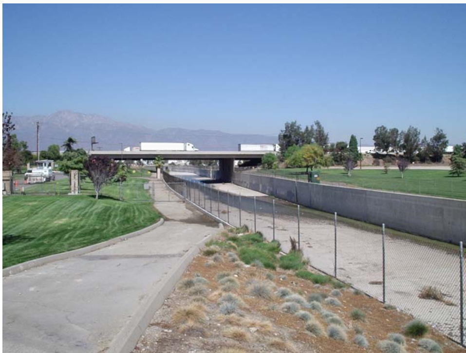
Figure 2 Photo of Cucamonga Creek at RP1 Survey Location
